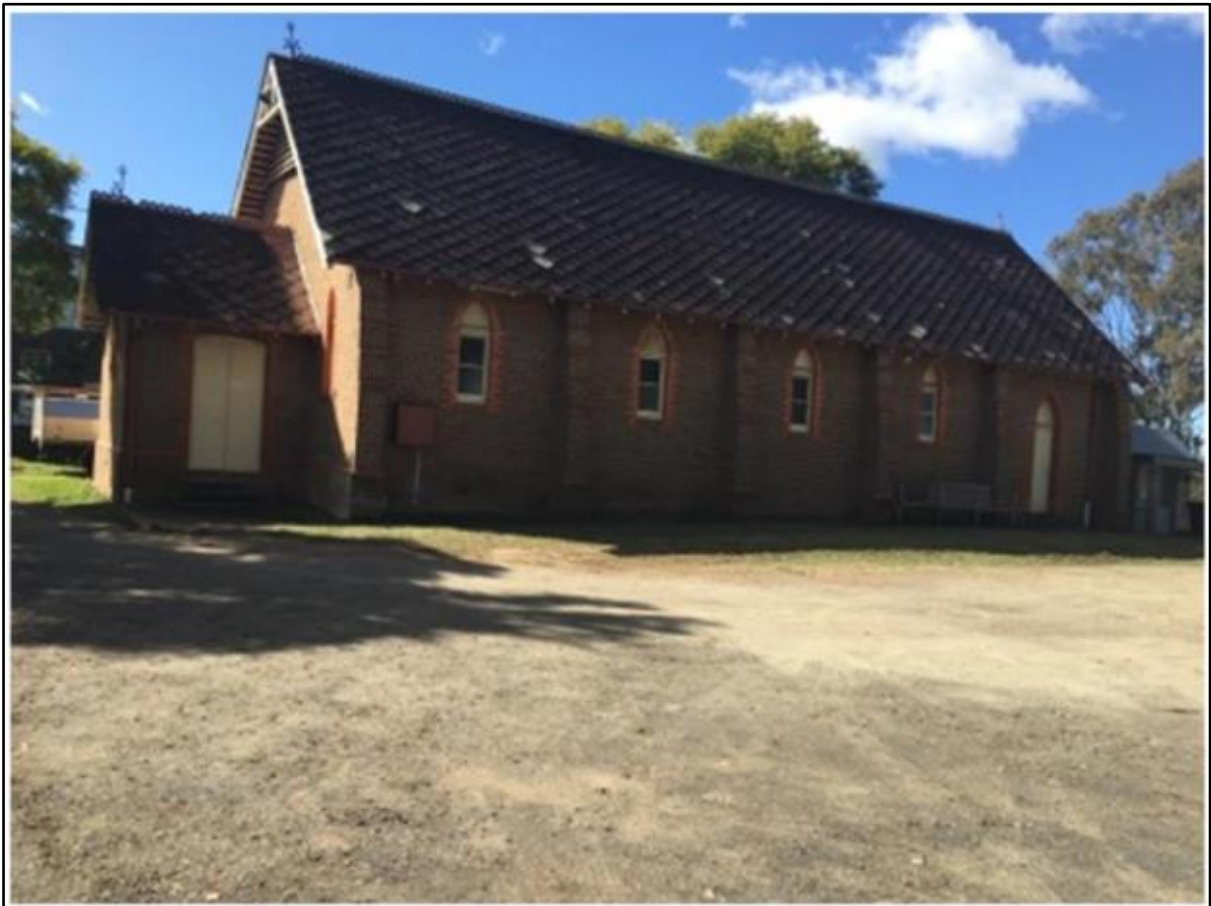
Figure 2 – View of western elevation of 1906 Church Hall
