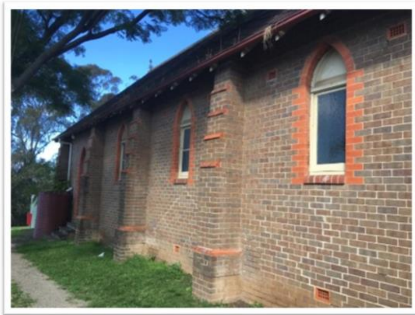
Figure 3 – View of eastern elevation of Hall
