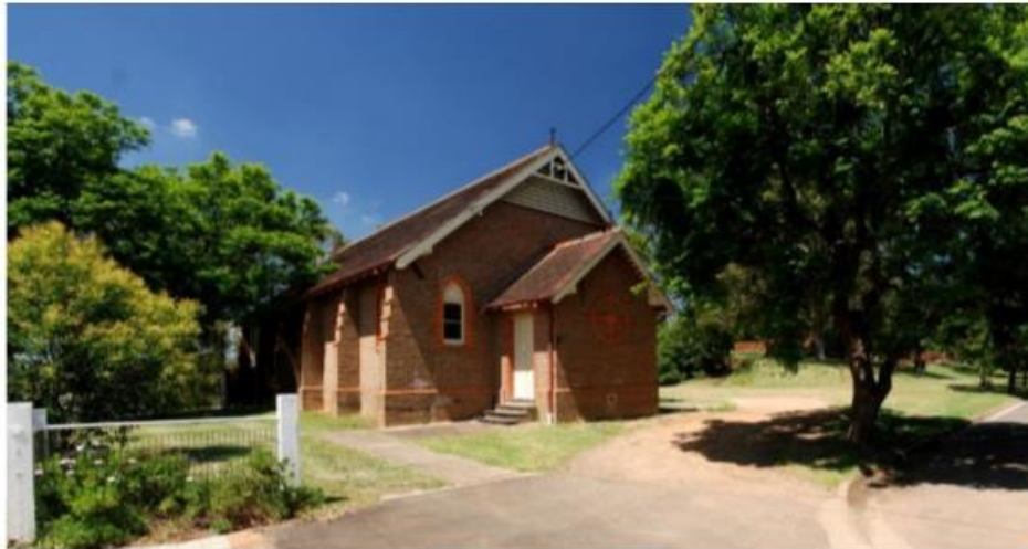
Figure 2: the 1906 Church Hall seen from Broughton Street, looking south-west.
