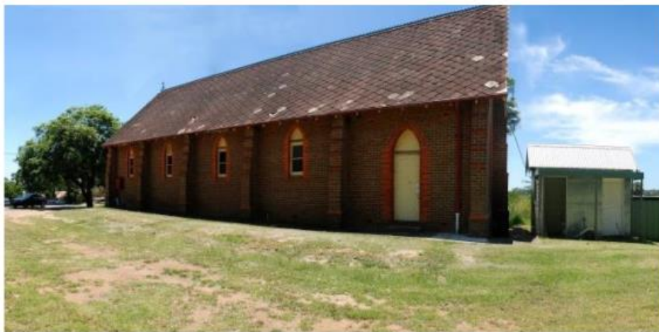
Figure 3: the west elevation of the Church Hall
