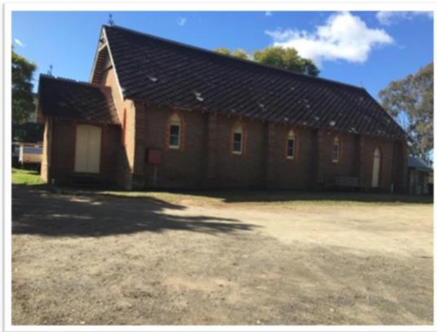
Figure 4 – View of western elevation of Hall
