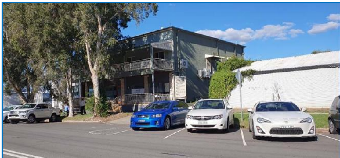
Figure 9: 16 Mitchell Street, Camden.
