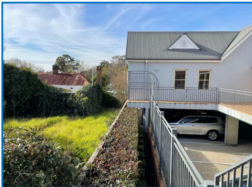
Figure 12: Boundary of the site looking east, toward Elizabeth Street, adjoining site 19 Elizabeth Street.
