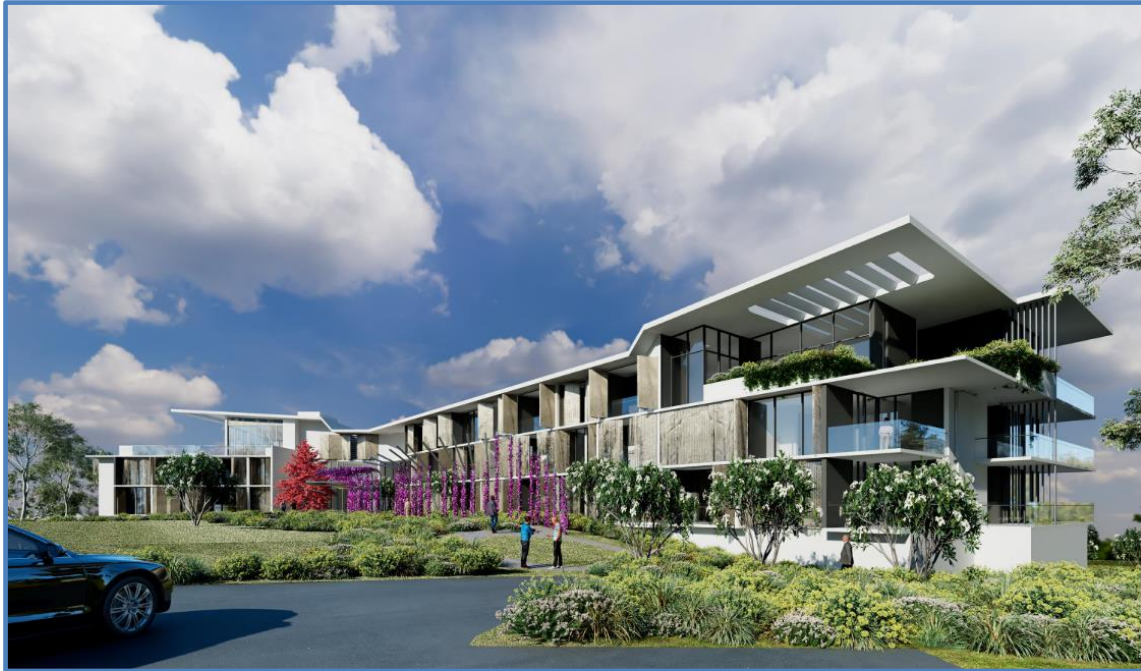
Figure 9: The proposed development as viewed from Mary Mackillop car park (facing east / viewed as figure 2).
