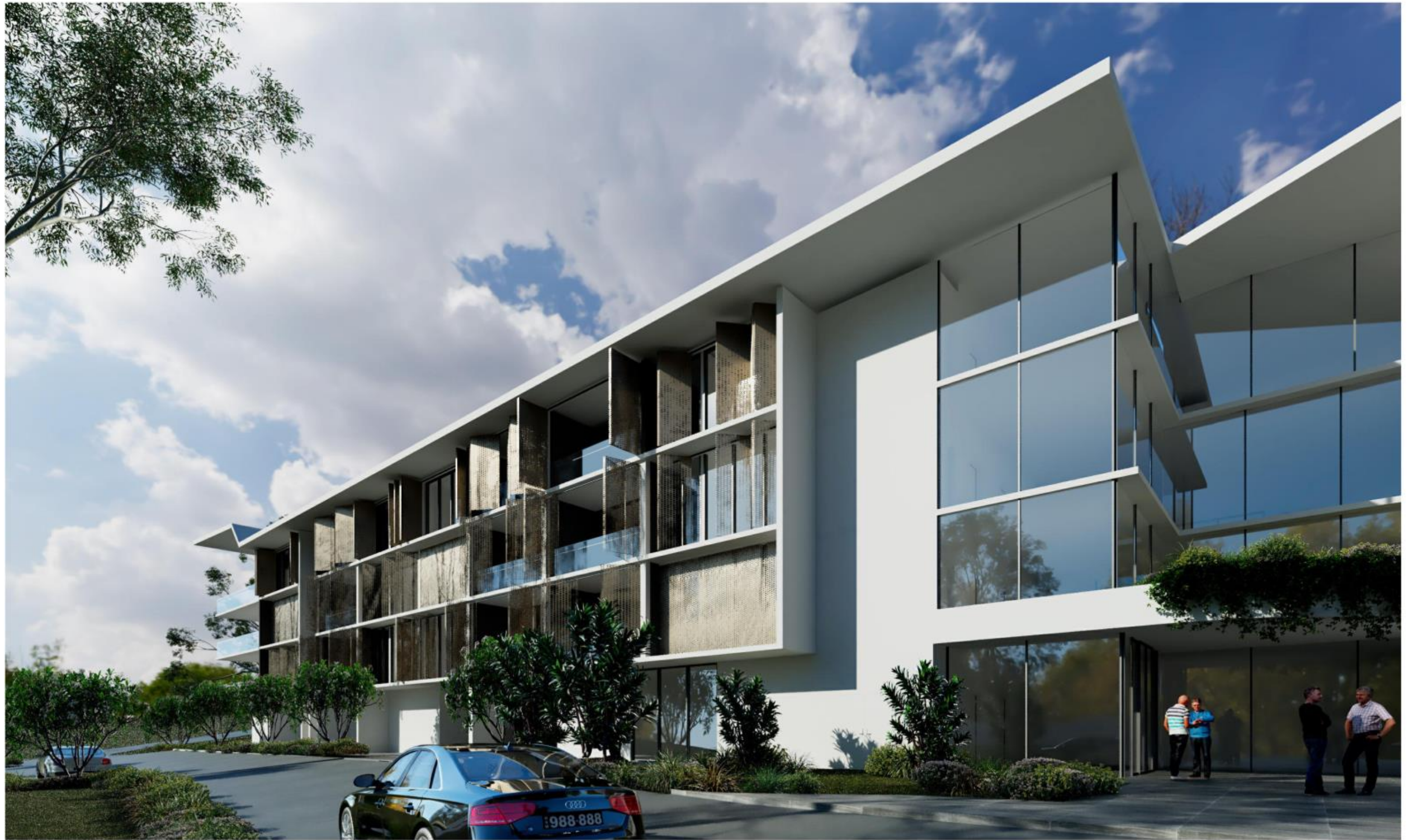
1 VIEW FROM SOUTH EAST LOOKING WEST ALONG MACKILLOP CIRCUIT (LOWER GROUND ENTRANCE RHS)
