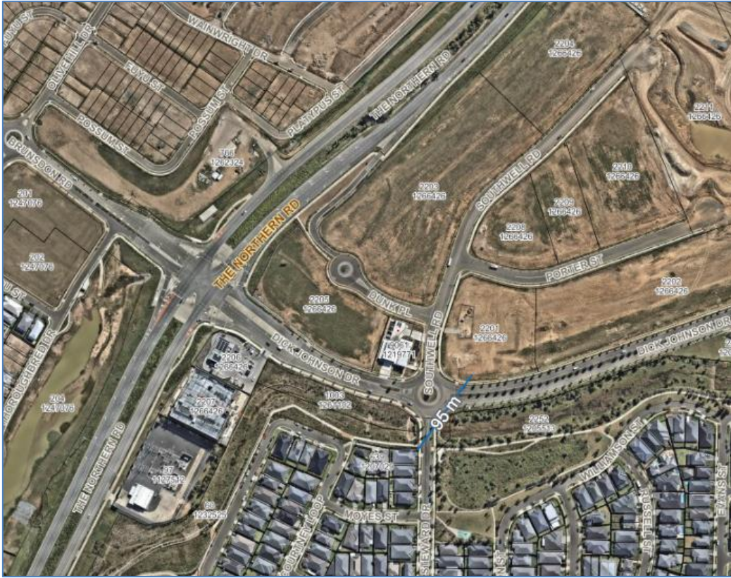
Figure 11: DA/2021/1220 located approximately 95m from residential lots.
