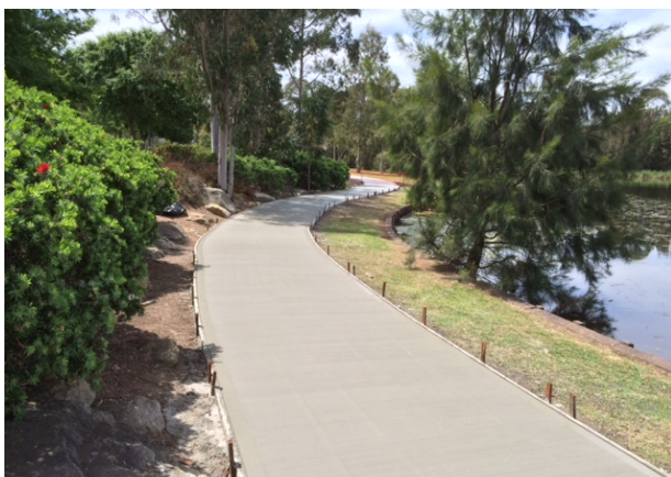
Harrington Park Footpath Construction
