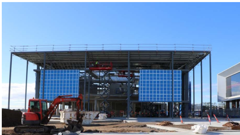
Construction of new Oran Park Library and Community Centre
