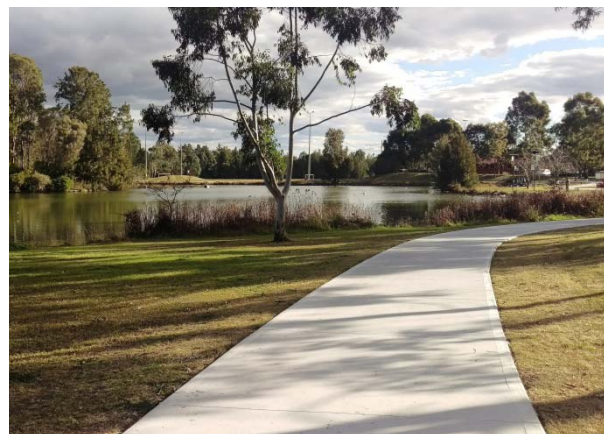
Harrington Park Footpath Construction Complete
