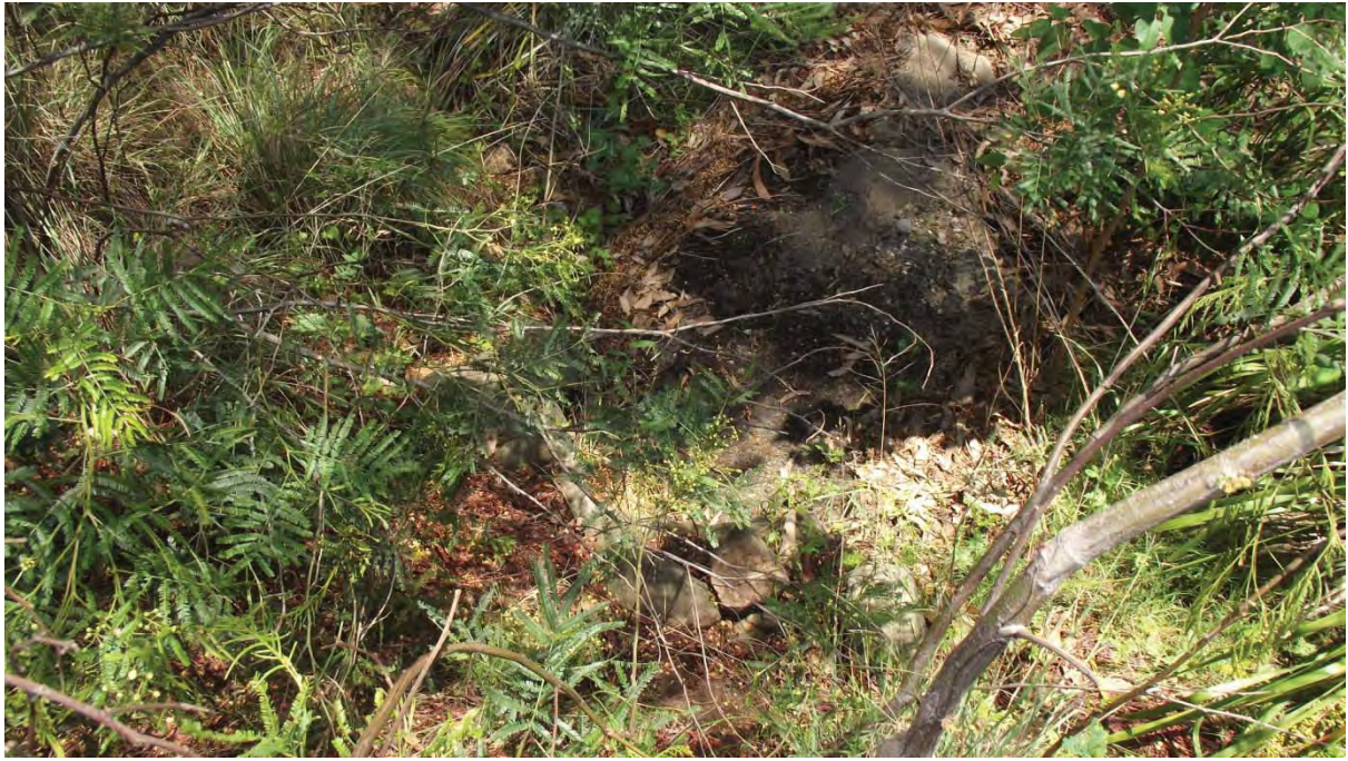
HEAD WALL AT DOWNSTREAM
