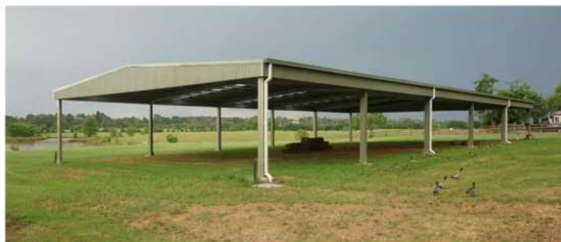
New Building - Covered Outdoor Working Area (COWA)
