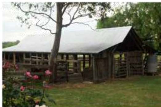
Barn after restoration
