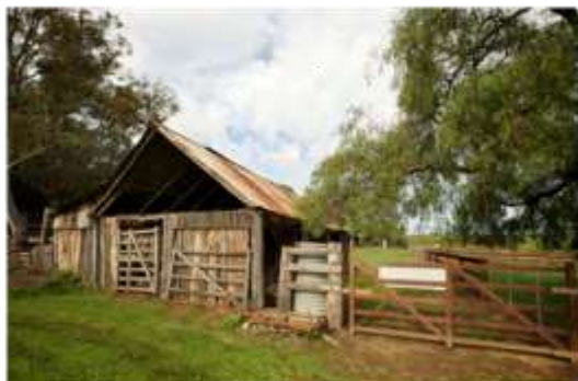
Barn before restoration
