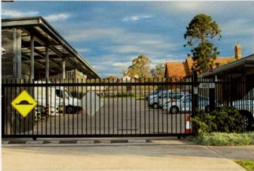
Figure 11 View corridors south through Police Station car park School Church and St Thomas Chapel. Showing the impact of high fencing and carport structure.
