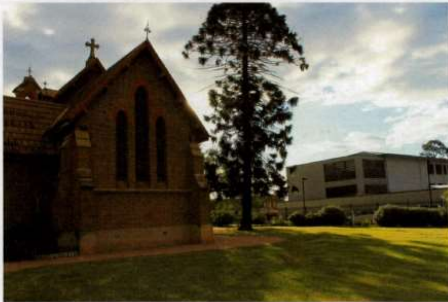
Figure 8 View corridors west of School Church towards St Thomas Chapel.
