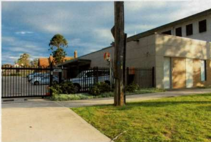
Figure 12 Close up of view corridors southwest through Police Station car park School Church and St Thomas Chapel.
