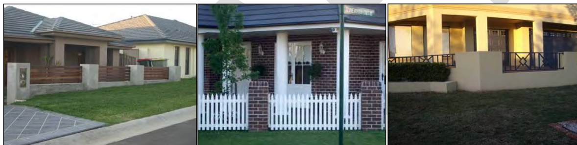
Front fencing with infill panels
