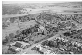
Aerial of Camden c. 1940
