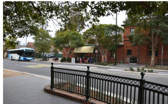
Paving, John Street
