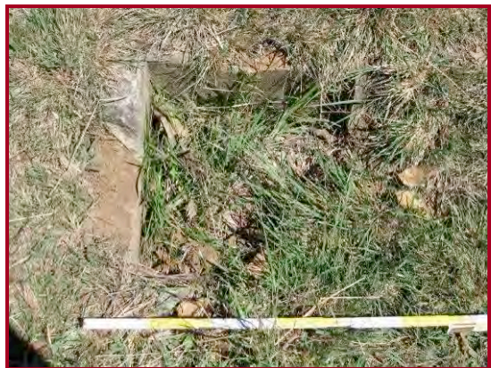
Figure 16. Gully trap near the cistern.
