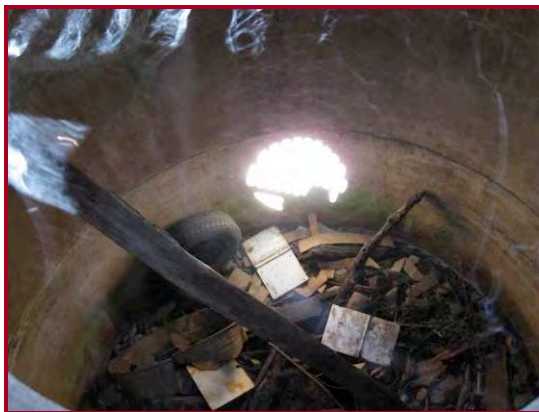
Figure 15. Interior of the cistern.
