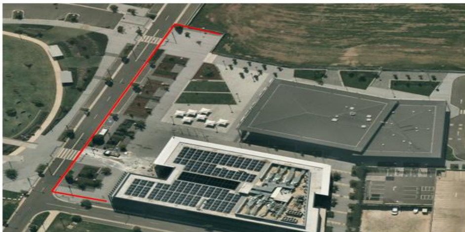
Figure 1: Various locations along the Oran Park Library and Administration Building Forecourts
