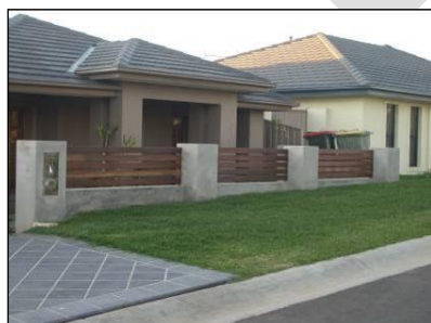
Front fencing with infill panels
