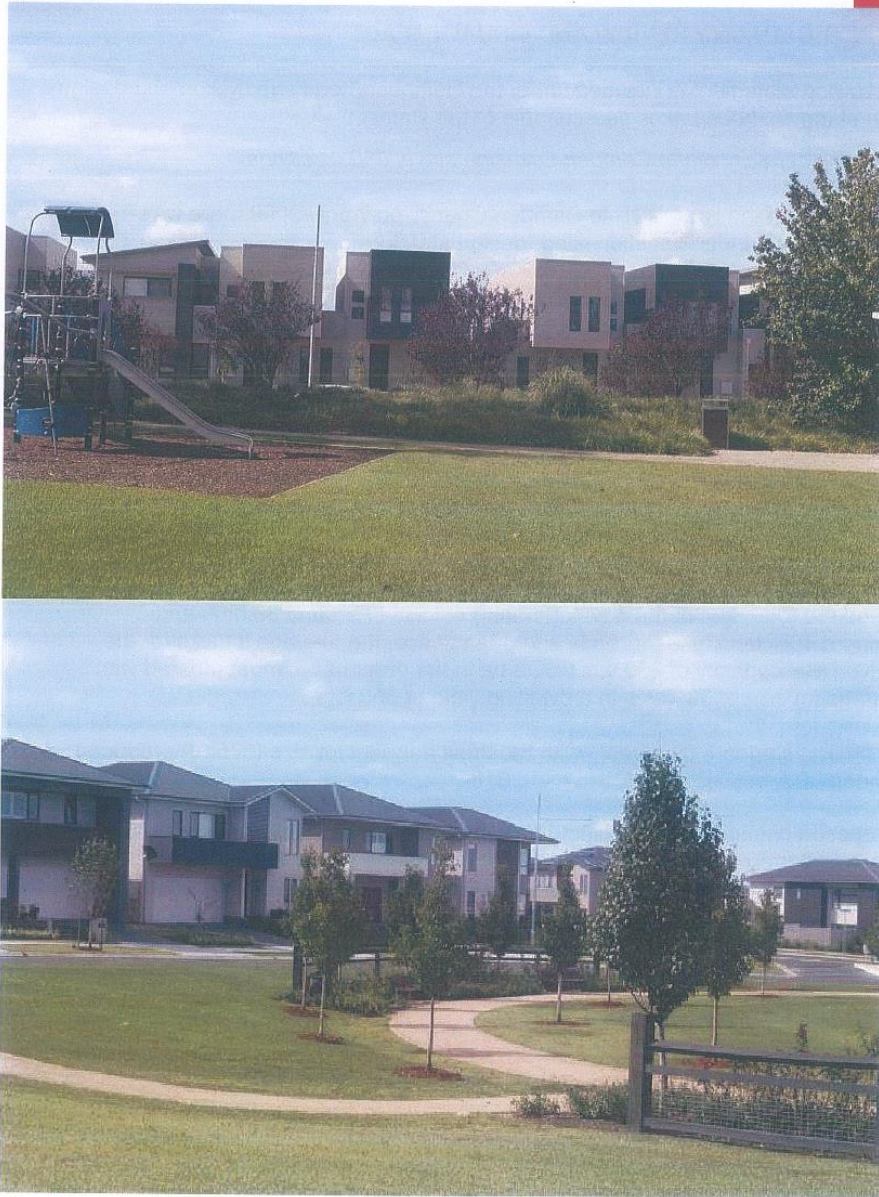
Figure 22 – Townhouses and 'standard' housing development at The Hermitage
