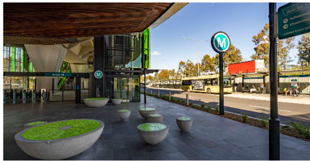
Figure 17 (bottom): Example of a Metro station Source: Transport for NSW
