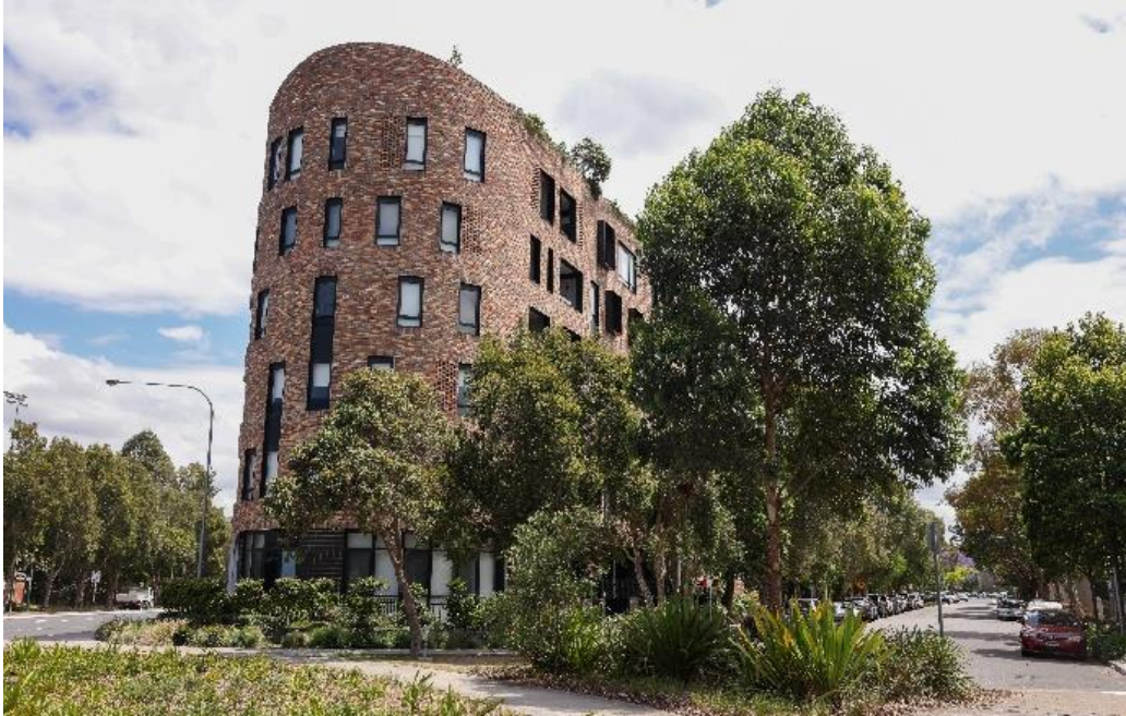
Figure 4: Residential flat building on Huntley Street, Alexandria
