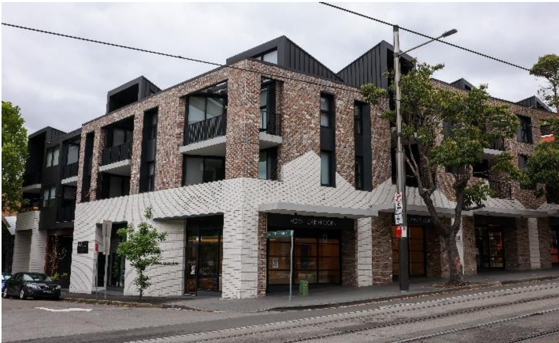
Figure 4: Shop top housing in Surry Hills
