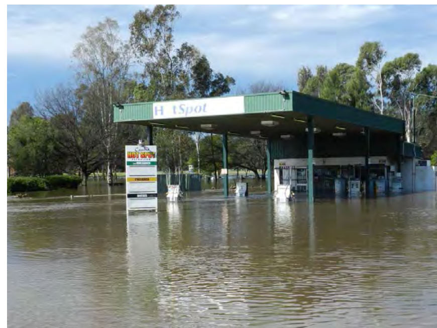
June Floods 2016 Cnr John Street & Camden Valley Way, Camden
