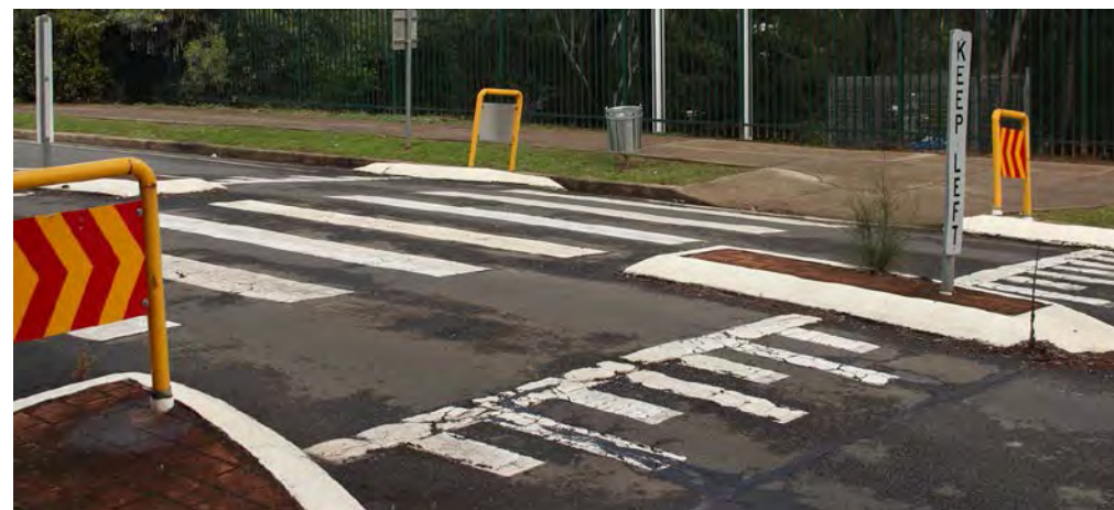
Pedestrian crossing on Stenhouse Drive, Mount Annan to receive an upgrade
