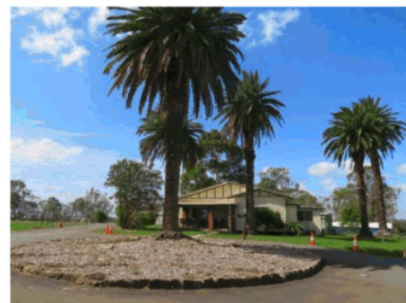
Figure 3.4 Turning circle in the centre of the site, with the interwar cottage in the background.
