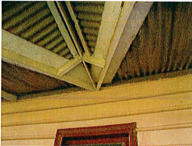
Detail of timber construction of gablet
