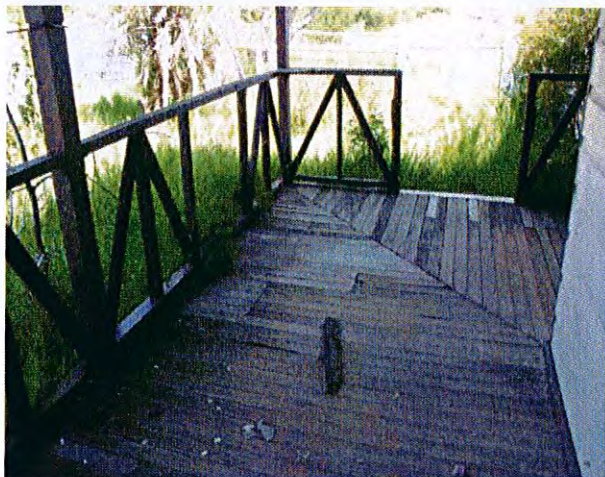
Western end of front verandah
