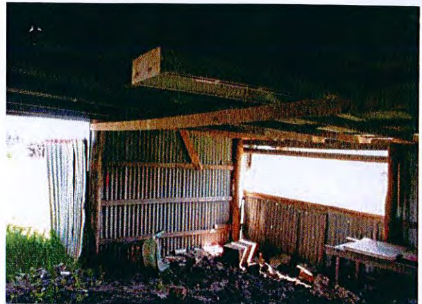
Internal space of the barn
