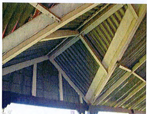
Detail of timber construction of the gablet
