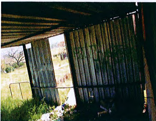
Aluminium cliplock material used for northern end of carport
