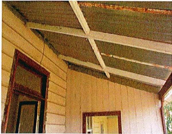
Detail of roof on eastern verandah
