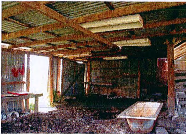
Interior space of barn
