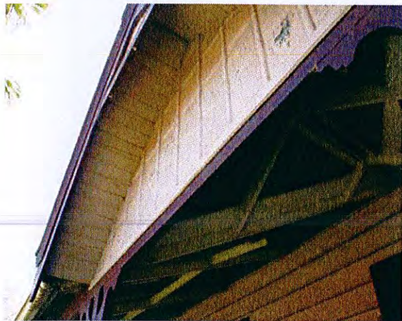
Detail of timber construction of the gablet
