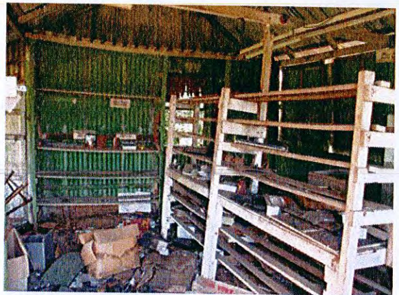
Internal layout of Building 6 showing timber pole construction and storage units
