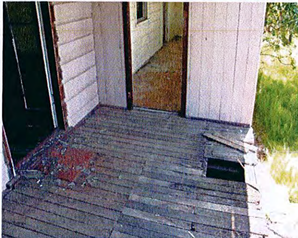
Floorboards to eastern verandah with Bedroom 4 at the northern end
