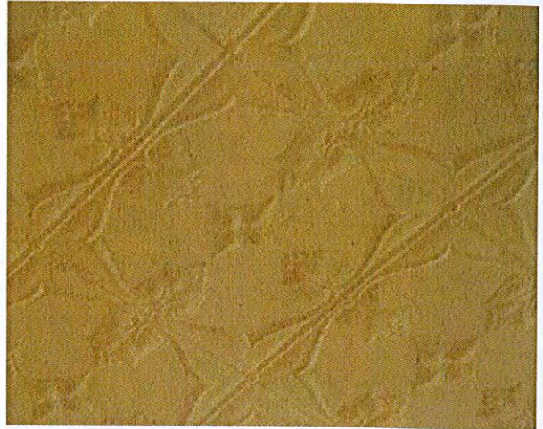
Detail of pressed metal ceiling
