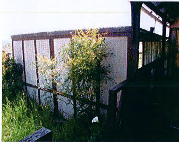
Southern wall of carport
