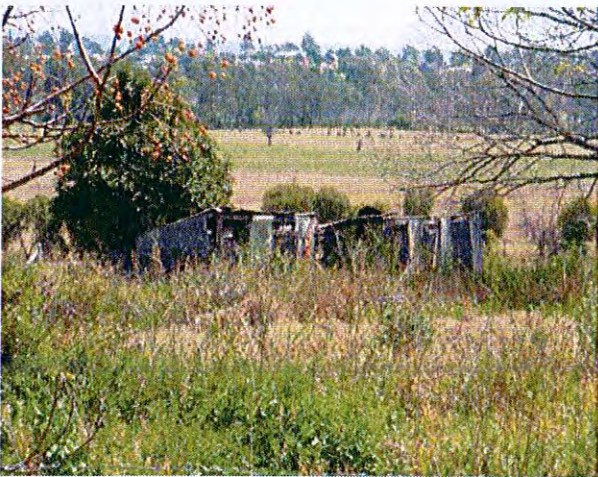
View from Building 8 to the northwest
