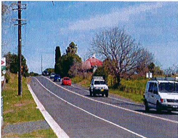
Yamba Cottage as viewed from the east along Camden Valley Way
