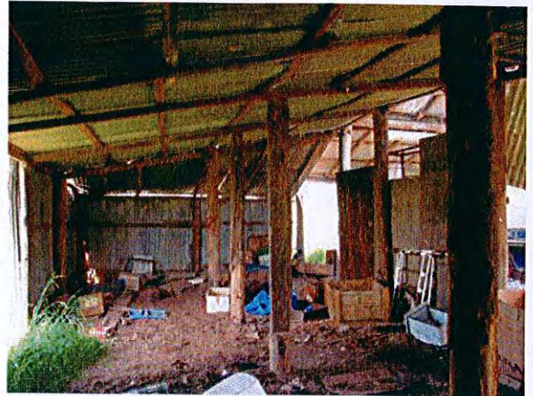
Lean-to section of Building 8
