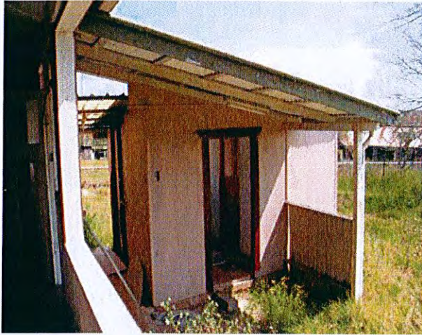
Structure 3 with open walled lean-to (Structure 4)
