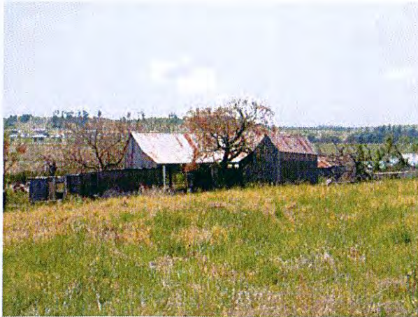
Buildings 8 + 9 as viewed from the the southwest.
