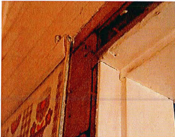
Original arched lintel removed from doorway to rear verandah
