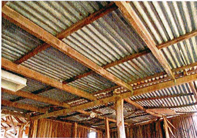
Detail of roof structure with timber frame and corrugated sheeting
