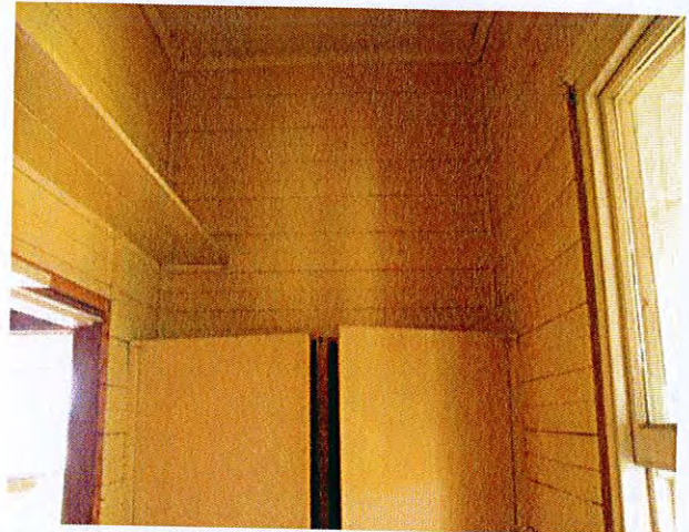
Tongue and groove walls in storeroom together with storage cupboard
