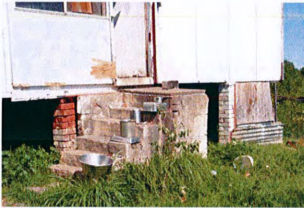
Brick piers and rendered concrete stairs to rear entrance
