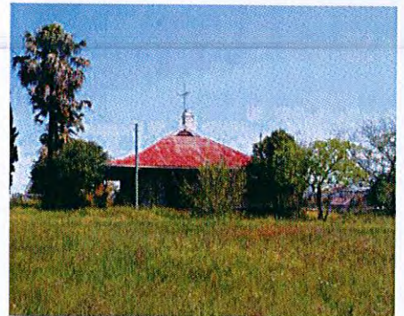
Eastern elevation showing gablet and masonry chimney
