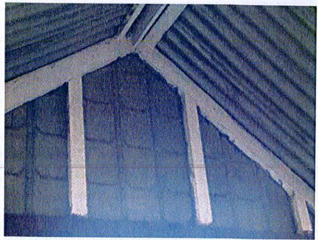
Corrugated roofing with proprietary pressed metal gable end
